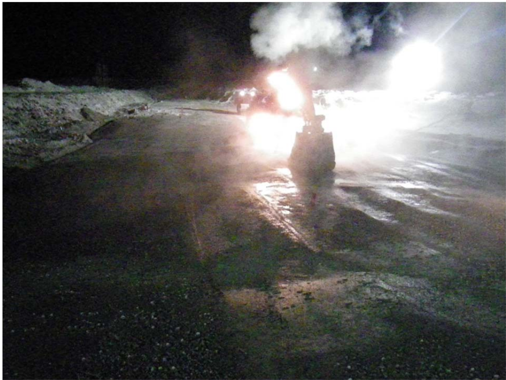
Photo 8: Cat 345 excavator placing FCM on nightshift.
