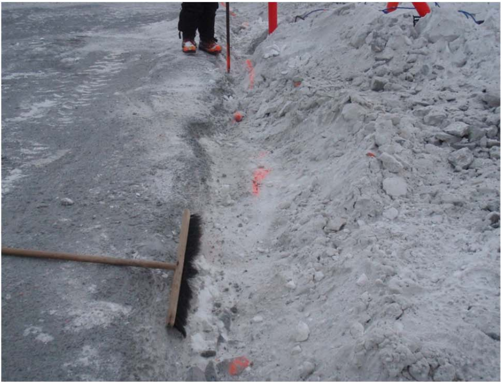
Photo 7: Area where additional snow clearing is required before core placement commences; approximately 0+95 looking southwest.
