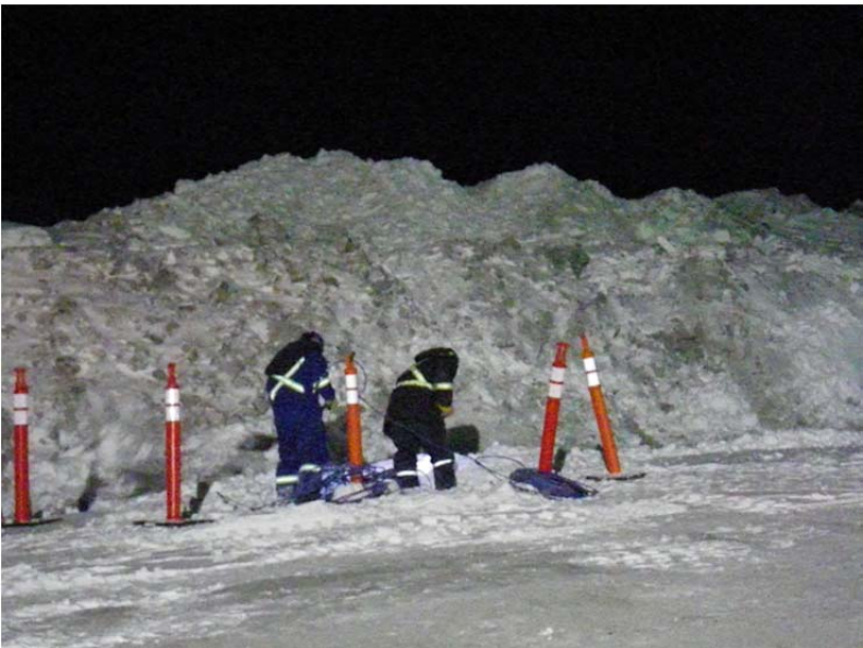
Photo 10: Labourers removing snow from around the thermistor cables.
