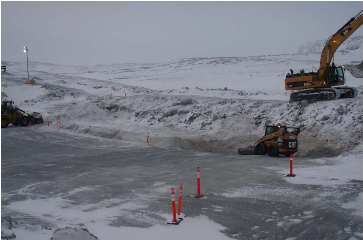
Photo 6: Downstream side of key trench snow clearing in preparation for core material placement.
