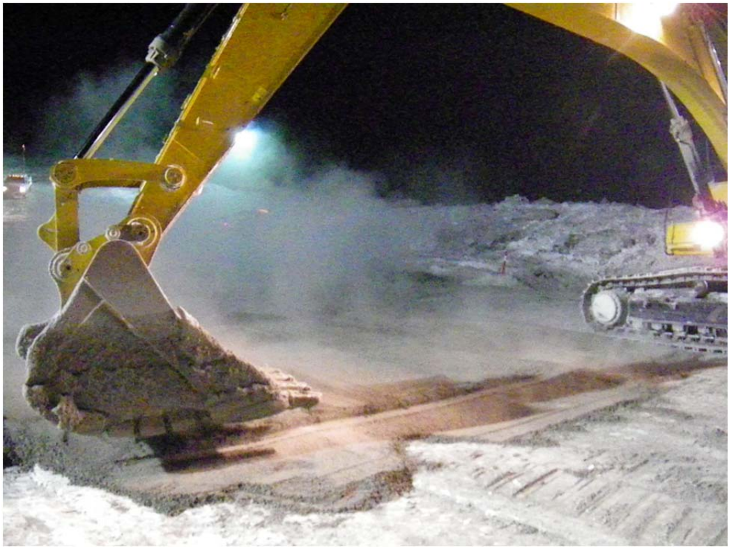
Photo 9: Excavator tying-in upstream edge with FCM.
